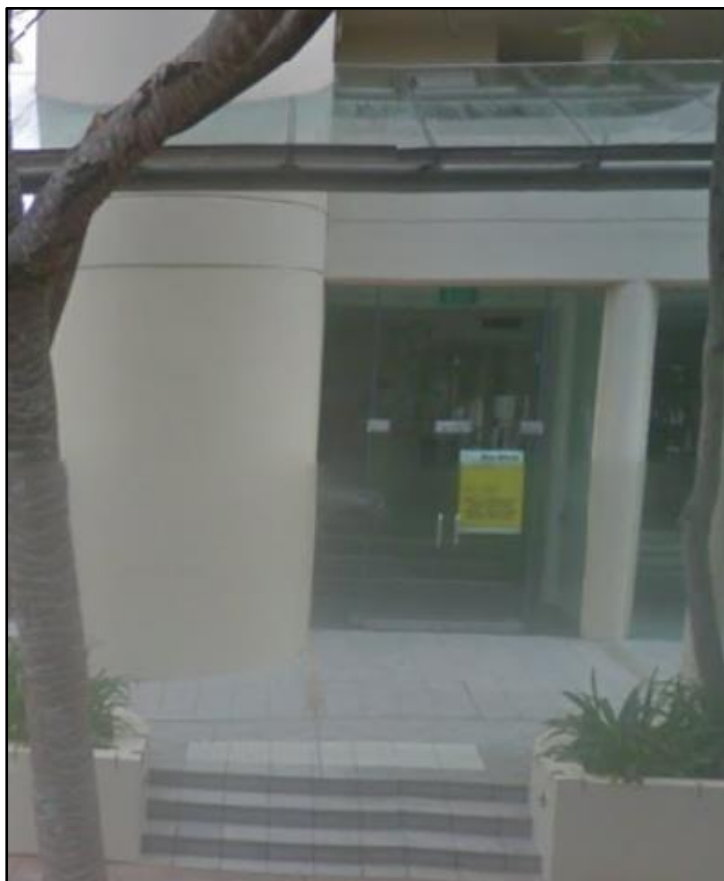
Figure 3 – The existing shop front
